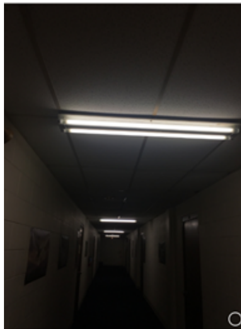
S Corridor Typical, fixtures are perpendicular and inadequate. Customer requests increased quantity with 8' LED Linear Strip Fixtures mounted Center-Parallel.
